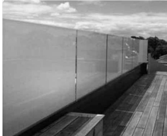
EXAMPLE FRAMELESS OBSCURED GLASS BALUSTRADE
